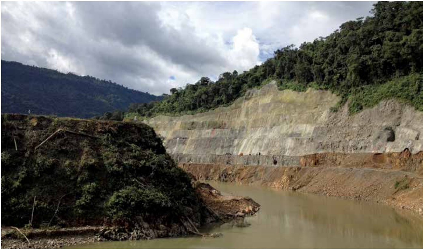
Construction scene of diversion dam in river.
